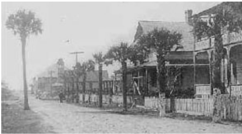
Palmetto Avenue, Pablo Beach, Florida looking east from what is currently the intersection of Beach Boulevard and 2nd Street. Photograph taken around 1906.
