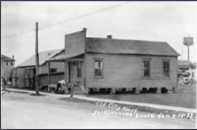
Photograph of the first City Hall built in Jacksonville Beach located on Pablo Avenue. Photo taken in 1927
